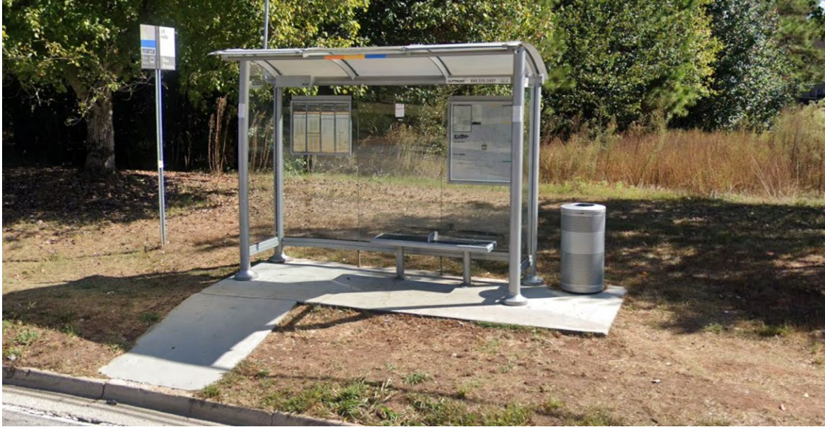
Figure 27 | Bus stop with all the desirable amenities...except for the sidewalk (Google Street View)
