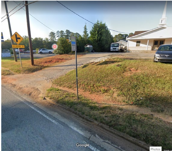
Figure 37 | Examples of various bus stops where informal pathways or waiting areas are etched into the dirt where a sidewalk or paved boarding area should be (Source: Google Street View)
